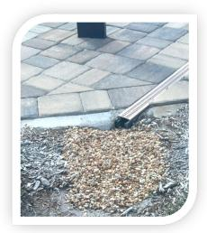
♣ The channel drain was causing minor erosion. Small river stones have been added to slow the water, stopping the erosion.
